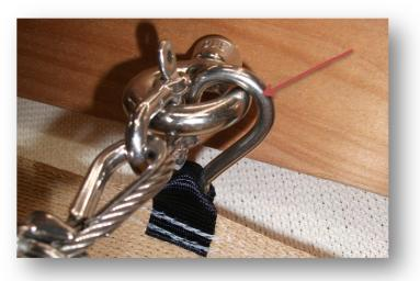
5. Install the cleat to tie the pull rope to when the sail is extended. (unless the option to use pulleys to retract/extended the sail is chosen)
